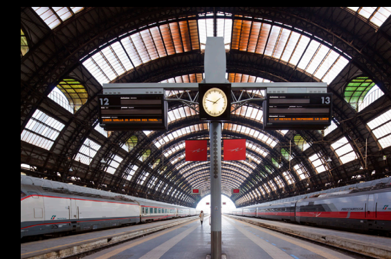
Milan Central Station (RFI property)
